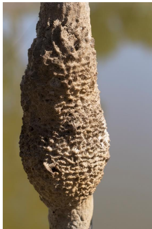
Freshwater sponge on pipe at Andrew's dam
