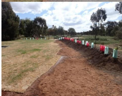
Completion of the Budyaan Baamirra Picnic Area works
