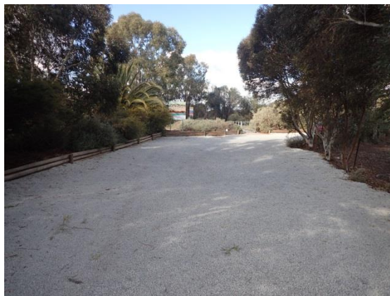
Upgraded Petersham Road Carpark.
